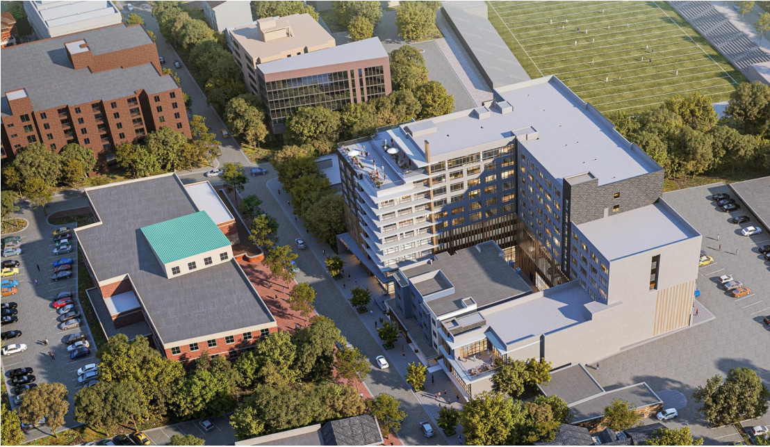
The State College Town Centre project, planned for South Allen Street
